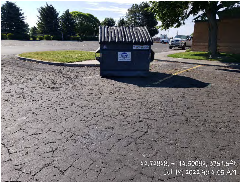
Northeast Corner of Building – Dumpster Area
