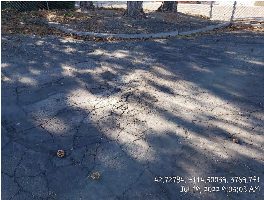
Southeast Corner – Undulating due to Tree Roots
