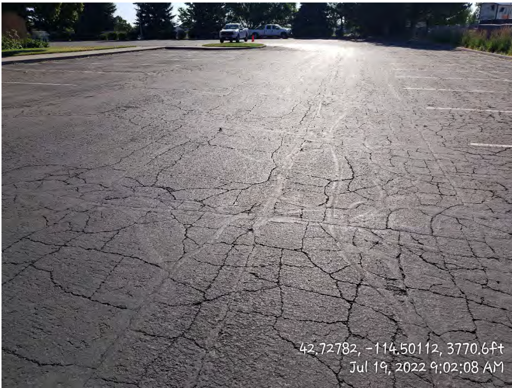
South of Building – Block and Alligator Cracking
