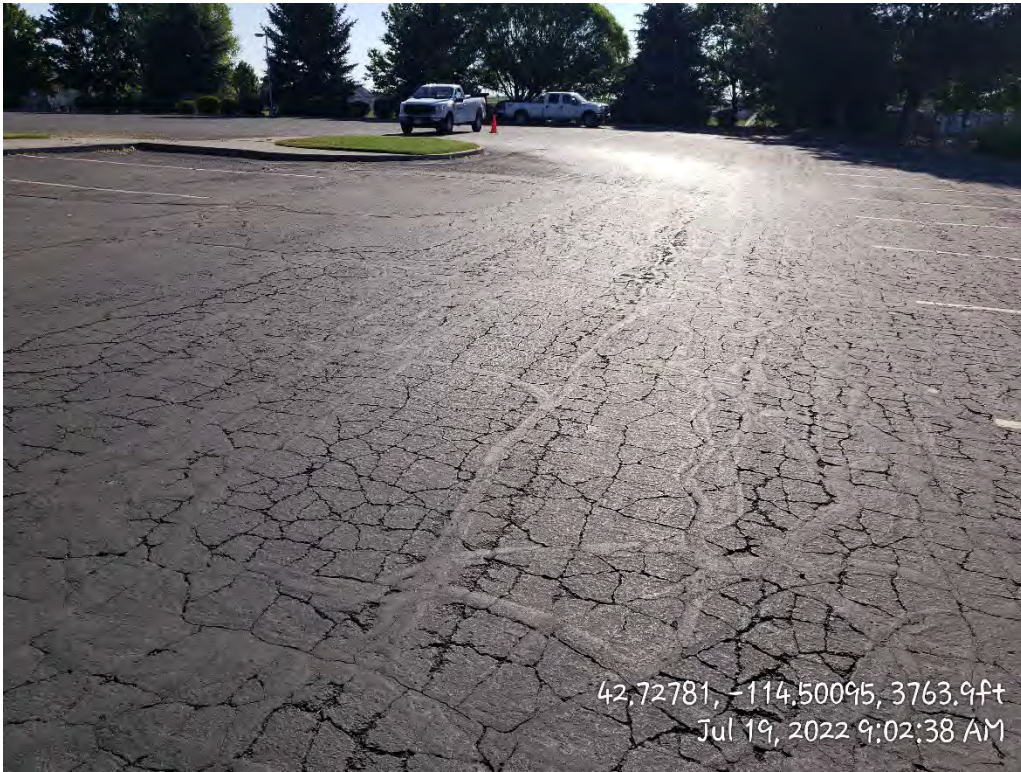
South of Building – Alligator Cracking
