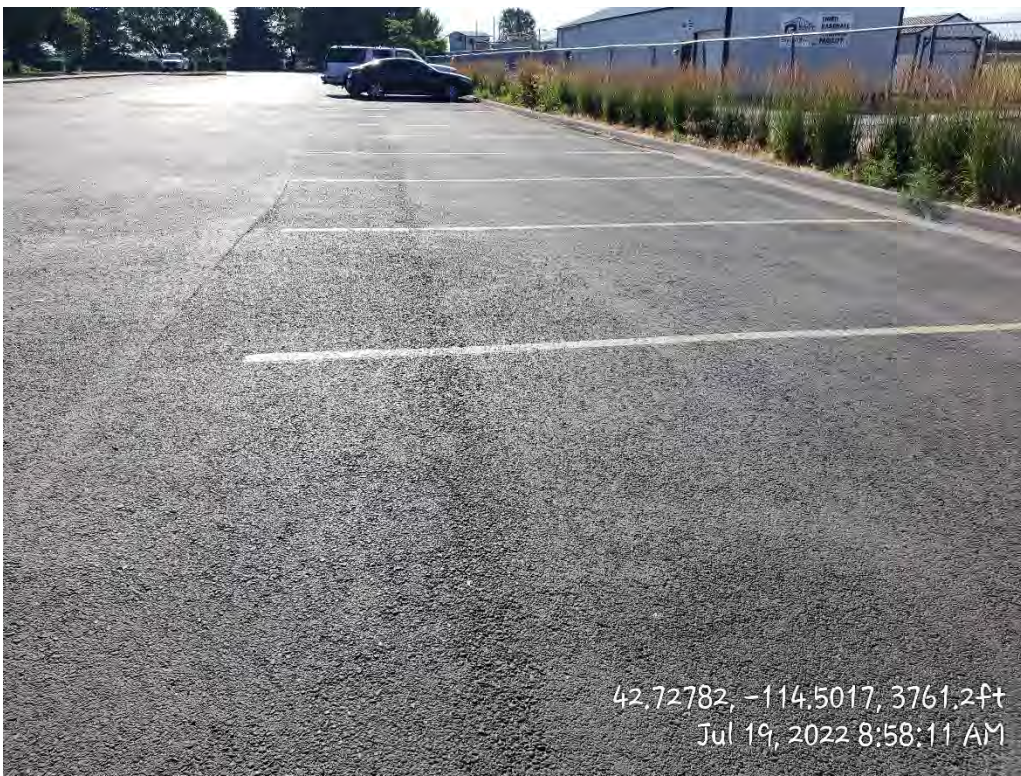
Southwest of Building – Few Visible Distresses
